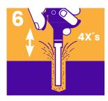
Blow out and remove all dust, dirt, debris, oil and any other contaminant from the control joint or crack. Use backer rod or kiln dried sand prior to application of adhesive.
